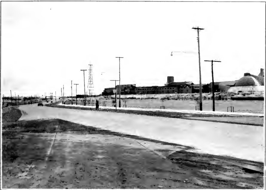
Concrete Pavement, Highway No. 67 at Timmins
